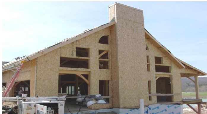
Hans Boxler's Hidden Valley Animal Adventure Construction underway
